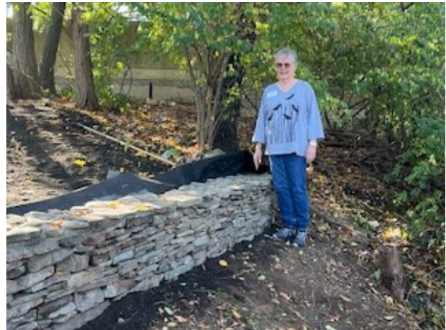
Carolyn in front of the new retaining wall
